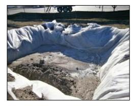
Plate 3-1 Typical concrete wash out areas
